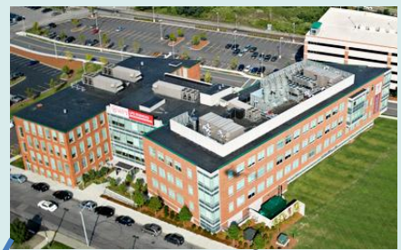
Gateway Park Life Sciences and Bioengineering Center
